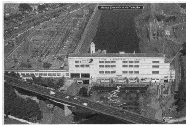
Fig. 2 Traição Pumped Storage Power Plant
