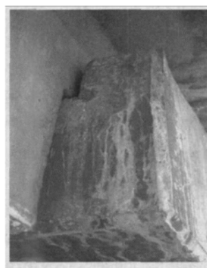
Fig. 3 Secondary beams of Beiyao cloverleaf junction
