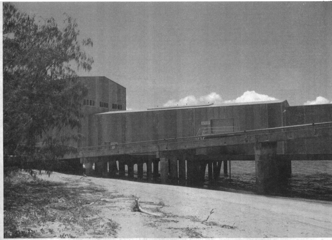
Fig. 2 View of Tail End Structure showing proximity to high water mark
